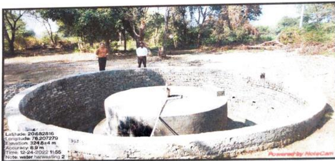
7.2/ 2: Roof Top Water Harvesting Near Borewell.
