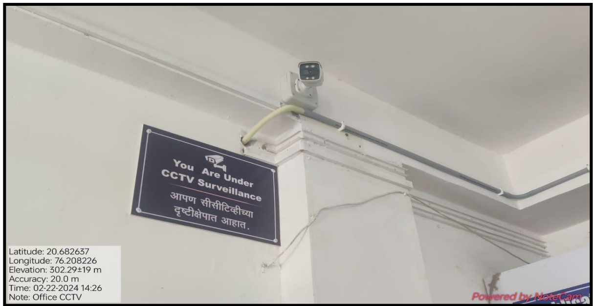
CCTV at Administrative Office
