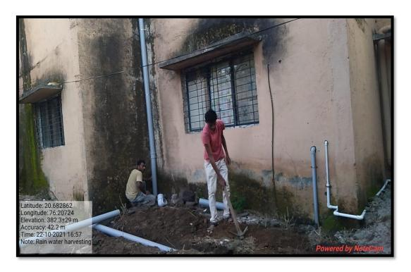
**PVC Pipes System for Roof Top Water Harvesting from Ladies Hostel**
