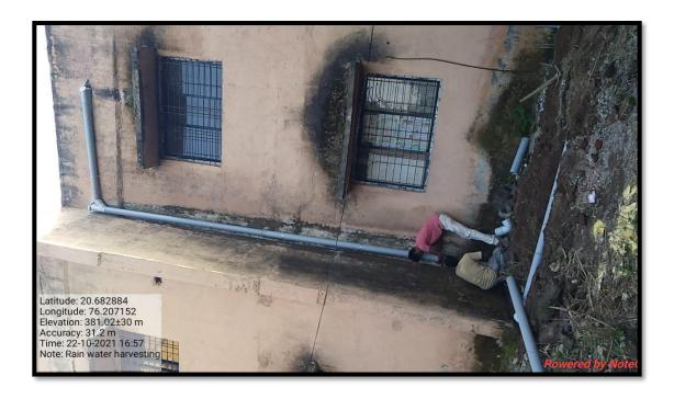
**PVC Pipes System for Roof Top Water Harvesting from Ladies Hostel**
