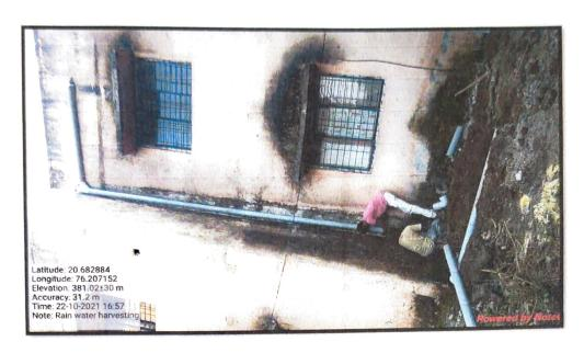
7.2/3: PVC Pipes System For Roof Top Water Harvesting.
