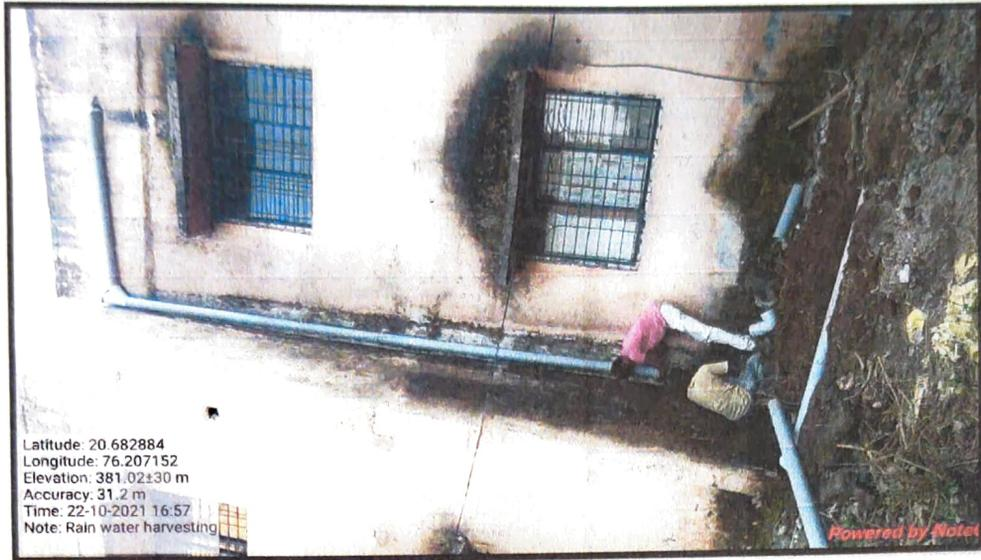
7.2/ 3: PVC Pipes System For Roof Top Water Harvesting.
